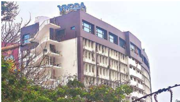
A view of the VMRDA Office in Visakhapatnam
