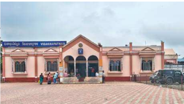
Gnanapuram railway station entrance which is set to be transformed Photos: Vasu Potnuru
