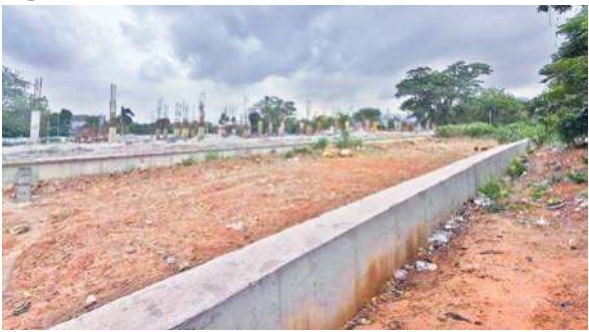
Additional platform works are in progress at Gnanapuram in Visakhapatnam
