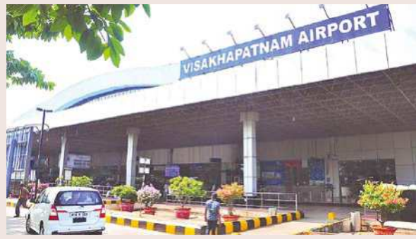
A view of Visakhapatnam Airport
