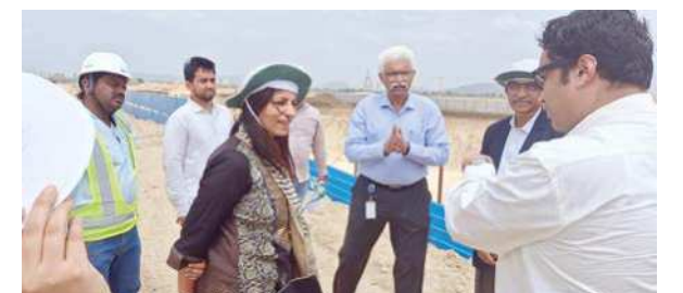
Gates Foundation India Country Director Archana Vyas at the construction site of the upcoming Basavatarakam Indo American Cancer Hospital at Thullur in Amaravati on Friday
