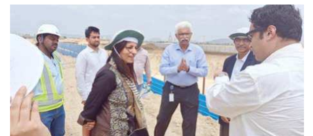
Gates Foundation India Country Director Archana Vyas at the construction site of the upcoming Basavatarakam Indo American Cancer Hospital at Thullur in Amaravati on Friday
