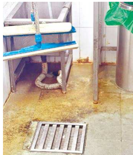
Unhygienic kitchen conditions observed during Food Safety Department inspections at food establishments
