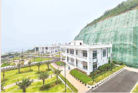
A view of the Rushikonda palace in Visakhapatnam
