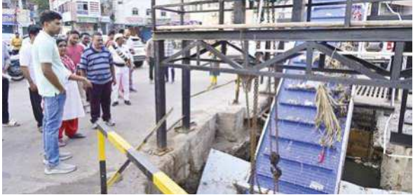
VMC Commissioner HM Dhyanachandra inspecting the ongoing desilting works at Krishnaveni Cloth Market on Tuesday
