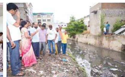
Satya Kumar Yadav inspecting an encroached drainage canal in Dharmavaram following recent rains and directing officials to take corrective measures
