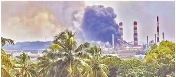
Smoke erupts after a loud explosion-like sound was reported from the MRPL premises near Jokatte in Mangaluru on Wednesday
