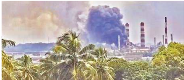
Smoke erupts after a loud explosion-like sound was reported from the MRPL premises near Jokatte in Mangaluru on Wednesday
