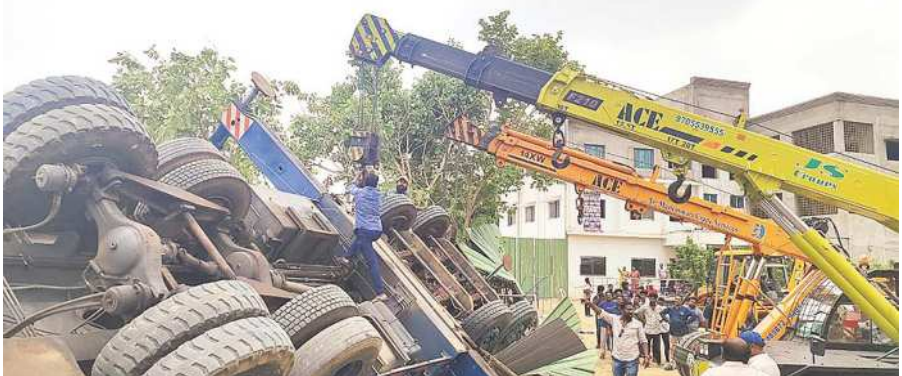
Efforts are underway to remove the crane from the pit in Tirupati on Tuesday
