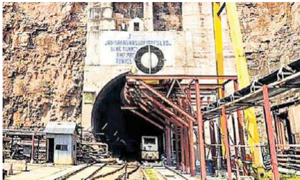
Tunnel 1, part of the SLBC, is a 43.93 km-long tunnel originating from the left bank of the Srisailem reservoir
