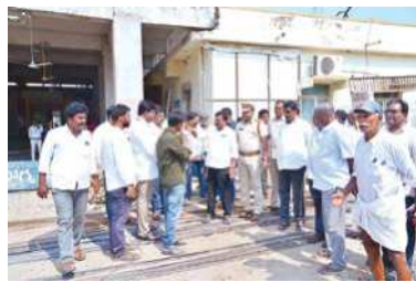
Minister DSBV Swamy inspecting renovation works of the PHC in Kondapi on Wednesday
