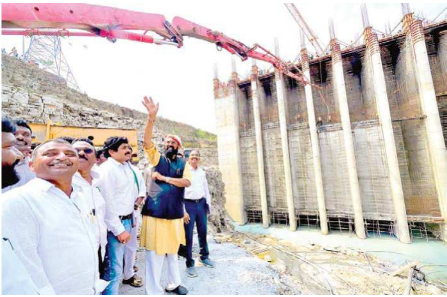
Minister Uttam Kumar Reddy along with officials examining Jawahar Janpahad lift irrigation project works
